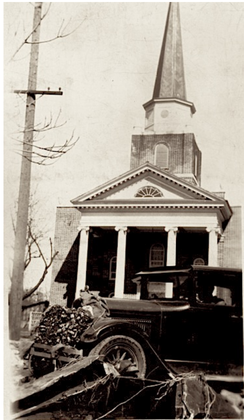
A view of First Congregational Church showing the aftermath of the March 1931 flooding of Mill Creek. Author's photo.
